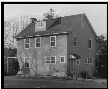
First parsonage (11 Saxer Ave.) demolished to build Epworth
